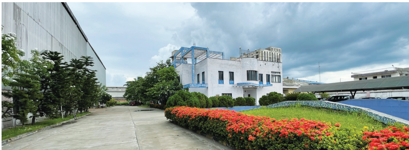
Electro Zavod factory
