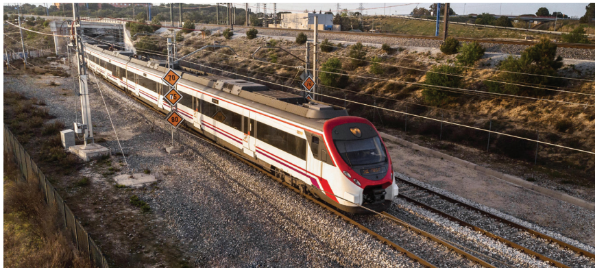
While VB train was cleared for 160 kph speed, proliferation of tracks to support this speed has not happened.
