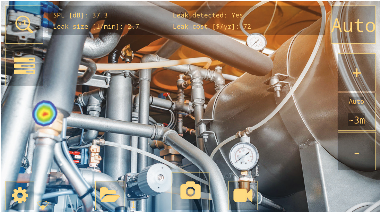
Industrial compressed air leak, as seen by the FLIR Si2-LD.
