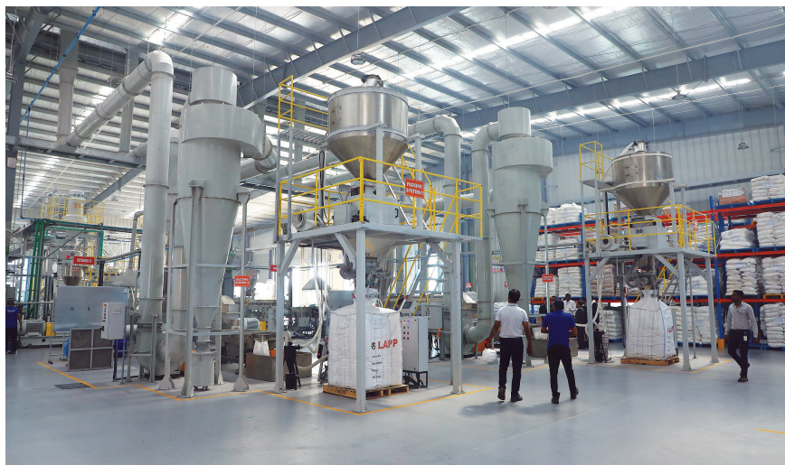
LAPP's new compounding plant at Bhopal
