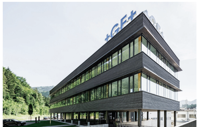
Georg Fischer Casting Solutions with the Altenmarkt site
