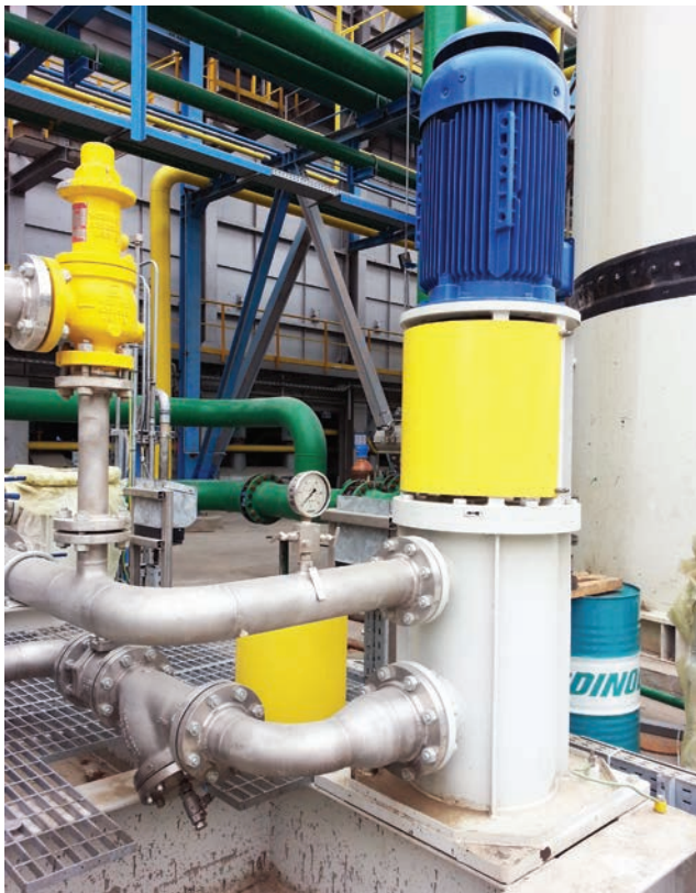
Plenty Triro rotary triple screw pumps from Celeros Flow Technology offer high-speed operation and compact design in a low cost, space saving unit.
