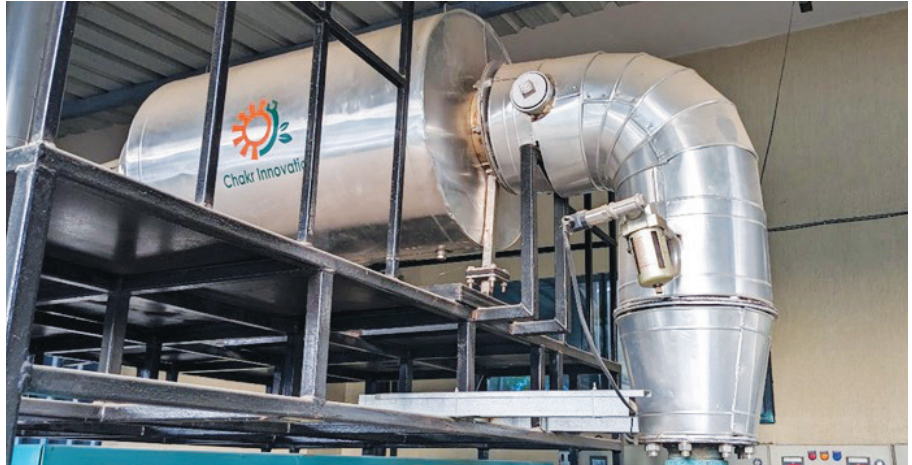
Chakr Shield: India’s first CPCB approved Retrofit Emission Control Device.
