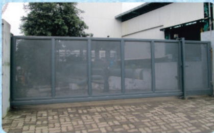
CANTILIVER SLIDING GATE
