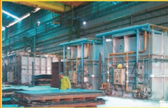
Gas Fired Rectangular Bell Furnaces
