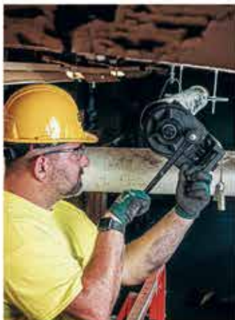
TEST PUMPS & GROOVERS
